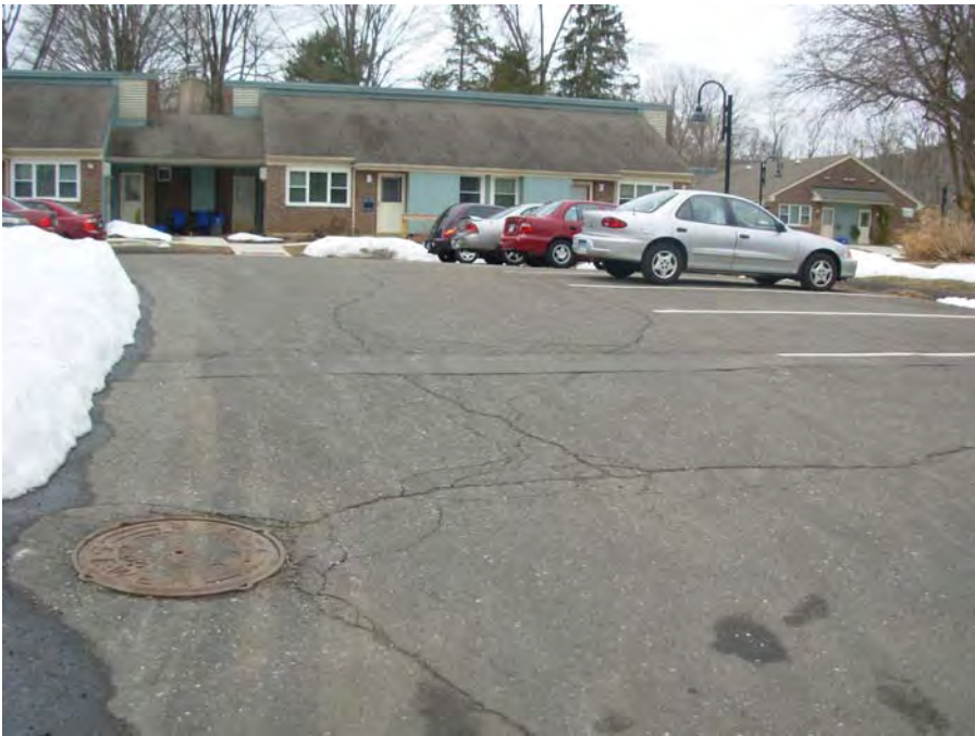
1. Parking area cracking and patched sections
