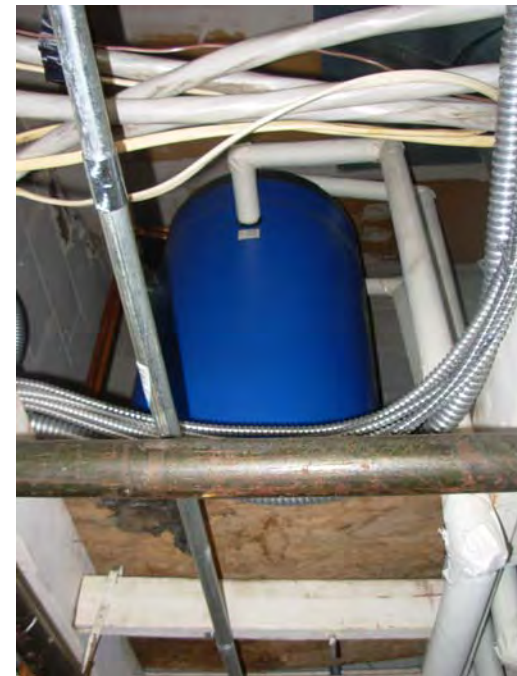
12. DHW heat exchanger - storage tanks
