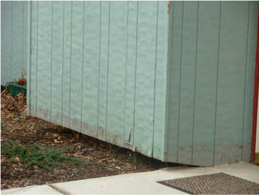
5. Spot deterioration of T1-11 siding
