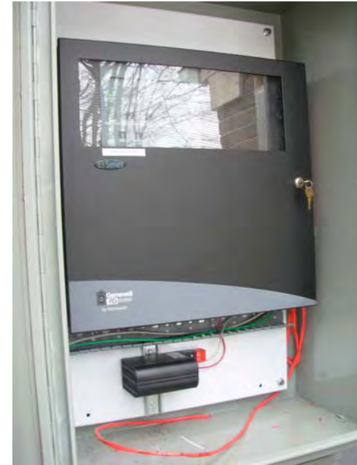
14. Fire detection and ECAS system monitoring panels
