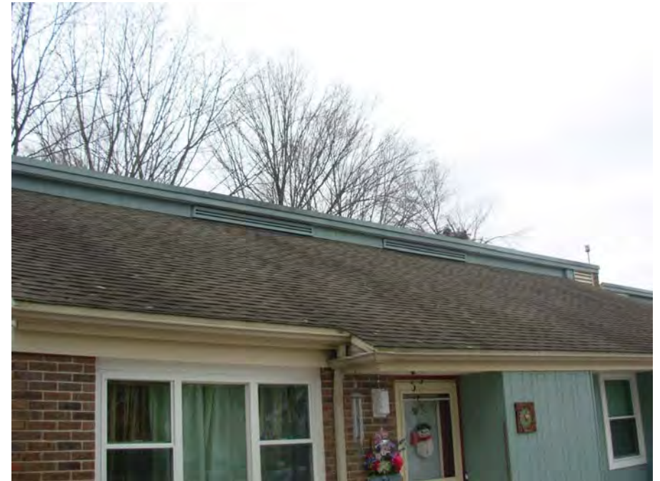
8. Roofing shingle staining, moss-lichen growth
