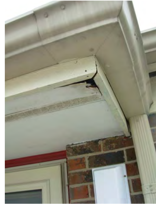
6. Spot deterioration of soffits and trim elements
